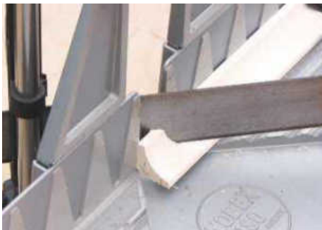
STEP 17. Add simple coving with 20mm scotia. Mark the front piece carefully and mitre the ends, pre-drilling holes to prevent splits
